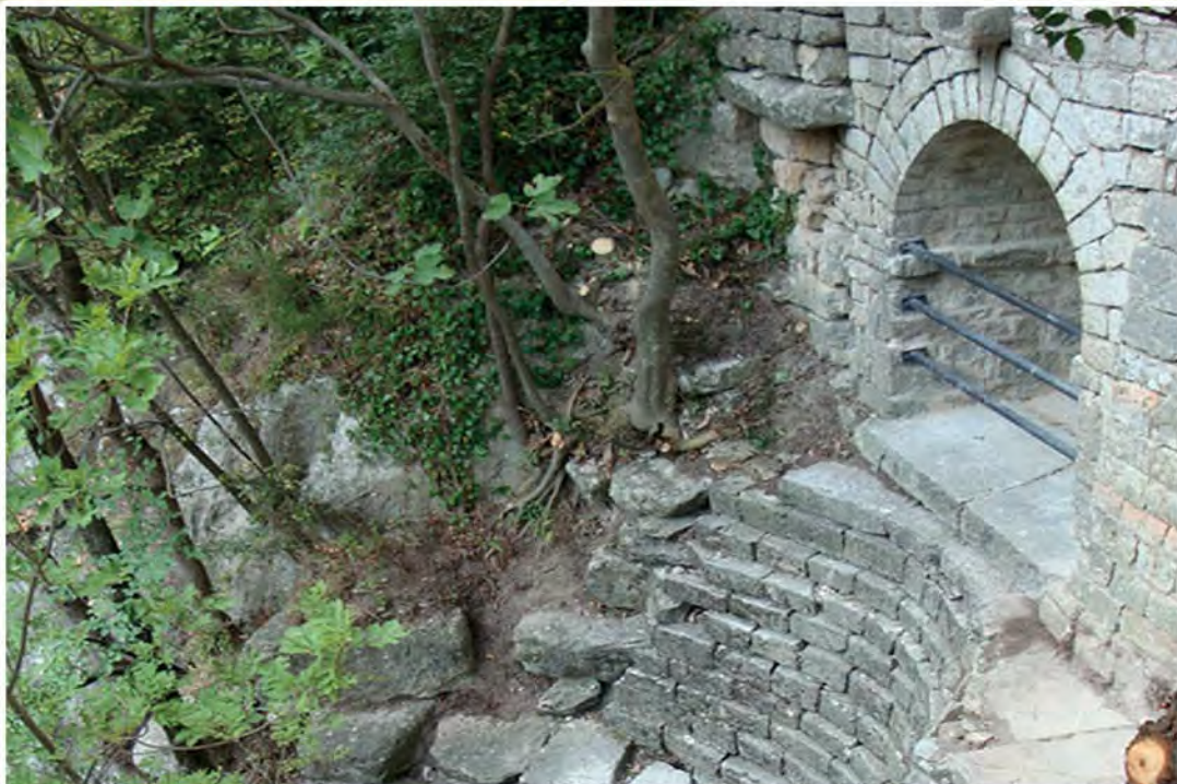
8 Uscita del chiaviccotto a valle. Output of the drainage channel downstream.
